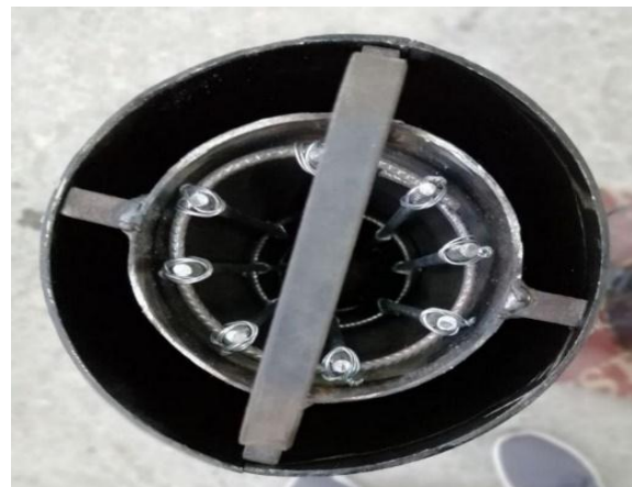
(c) Steel cage inside the mold
